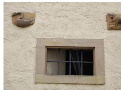
Detail Scheune (❶)
